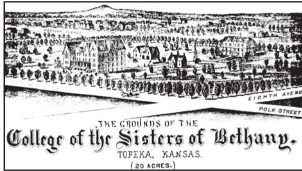
The College of the Sister of Bethany was located on 20 acres near downtown Topeka. This line drawing from the late 1800s shows its buildings, including the laundry (now the diocesan office) and barn (now the conference center).
